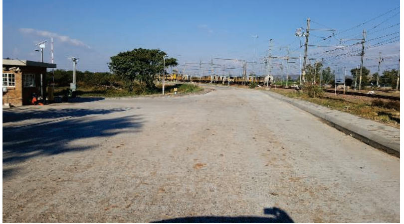
Hardstands & layerworks designed for forklifts & 30ton trucks.
